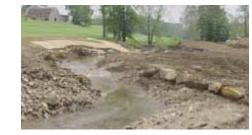
\* rock and log "toes" at the base of banks which are embedded with layers or mats of materials such as live branches and tree root "wads" for stability, and \* engineered bends or "meanders", "J's" or "V" vanes made of rocks or logs, riffle and pool sequences, and random boulder placement, all to slow stream flows.
